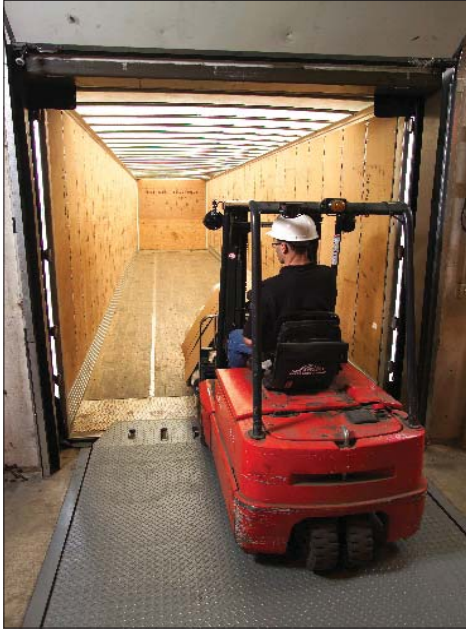
Exposed trailer door hinge gaps amount to 2.5 ft 2 of open space through which heating or cooling energy escapes.
